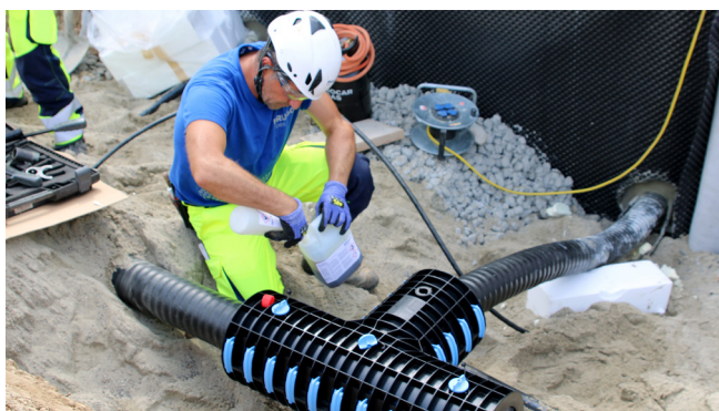
CALPEX clip shells provide perfect protection for junctions and connections underground.
